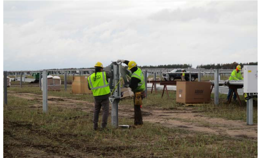
Gear and rack installation
