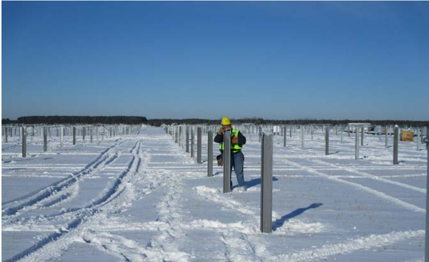
Inspecting pile placement
