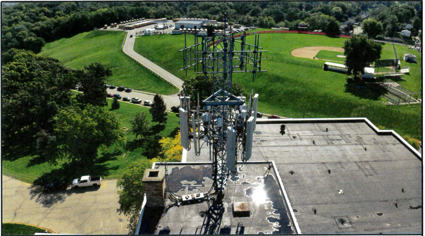
VIEW SOUTHEAST TOWARD PROJECT LOCATION
